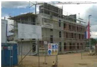
Construction of 40 apartments Knin, Croatia
