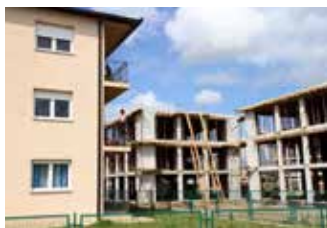
Construction of 120 apartments Konik Camp, Montenegro
