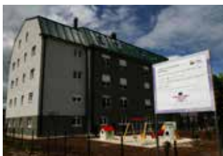
Construction of 62 apartments Niksic, Montenegro
