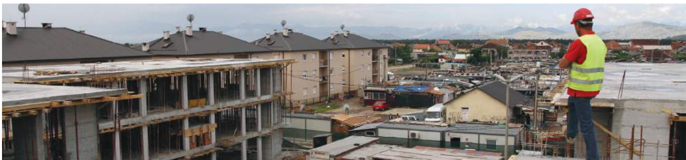
Construction of buildings at Konik Camp, Podgorica, Montenegro
